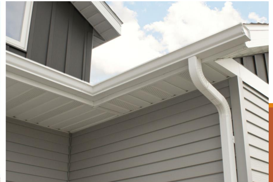
Eaves Protected by Soffit
